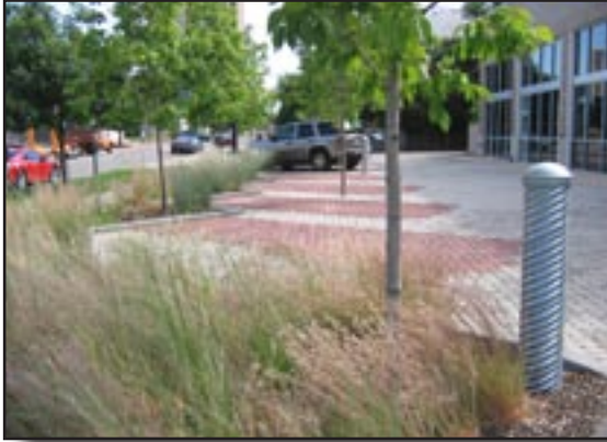
Porous pavers used in parking lot
