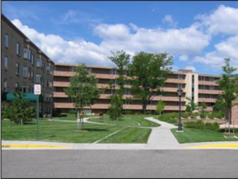
The sidewalk, adjacent to reinforced turf, doubles as an emergency vehicle access.
