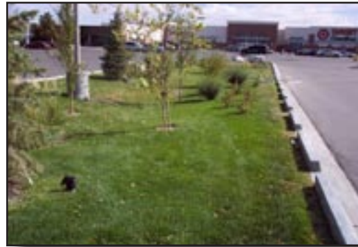
Parking lot "sumps," appropriately called porous landscape detention or rain gardens, are part of the parking lot design at the Aurora Super Target store, near Buckingham Plaza.
