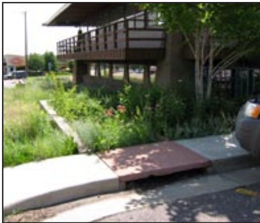
Parking lot runoff at Western Resource Advocates building in Boulder is directed to porous landscaped areas.
