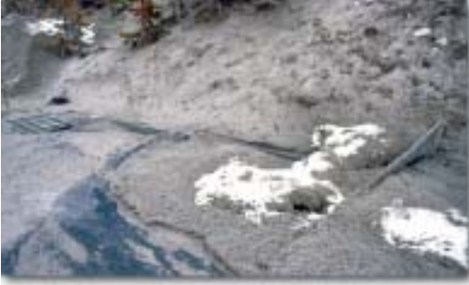
Material build up behind check dams
