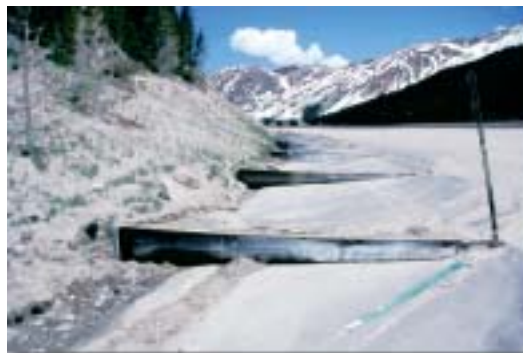
Check dams along Interstate 70
